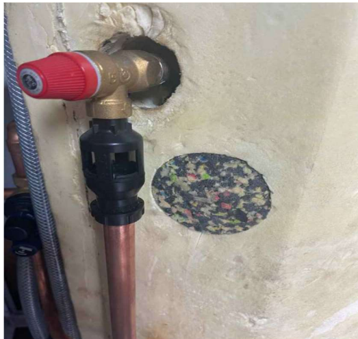
5. Cylinder Pressure Relief Valve & Tundish
